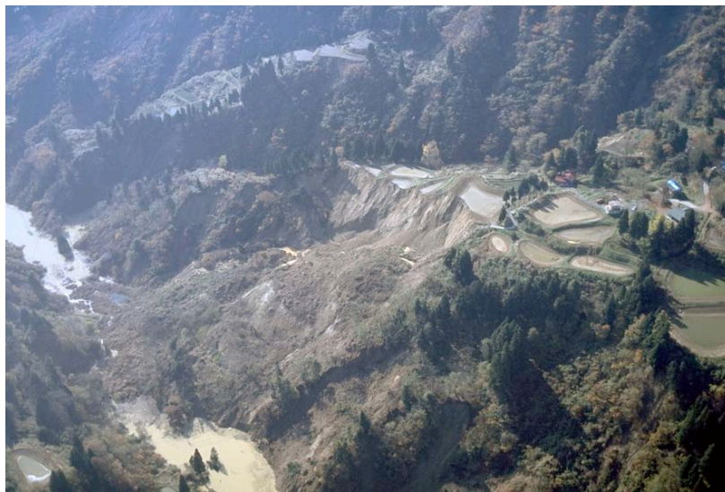
Pic.5 Landslide due to the Mid-Niigata earthquake 2004
